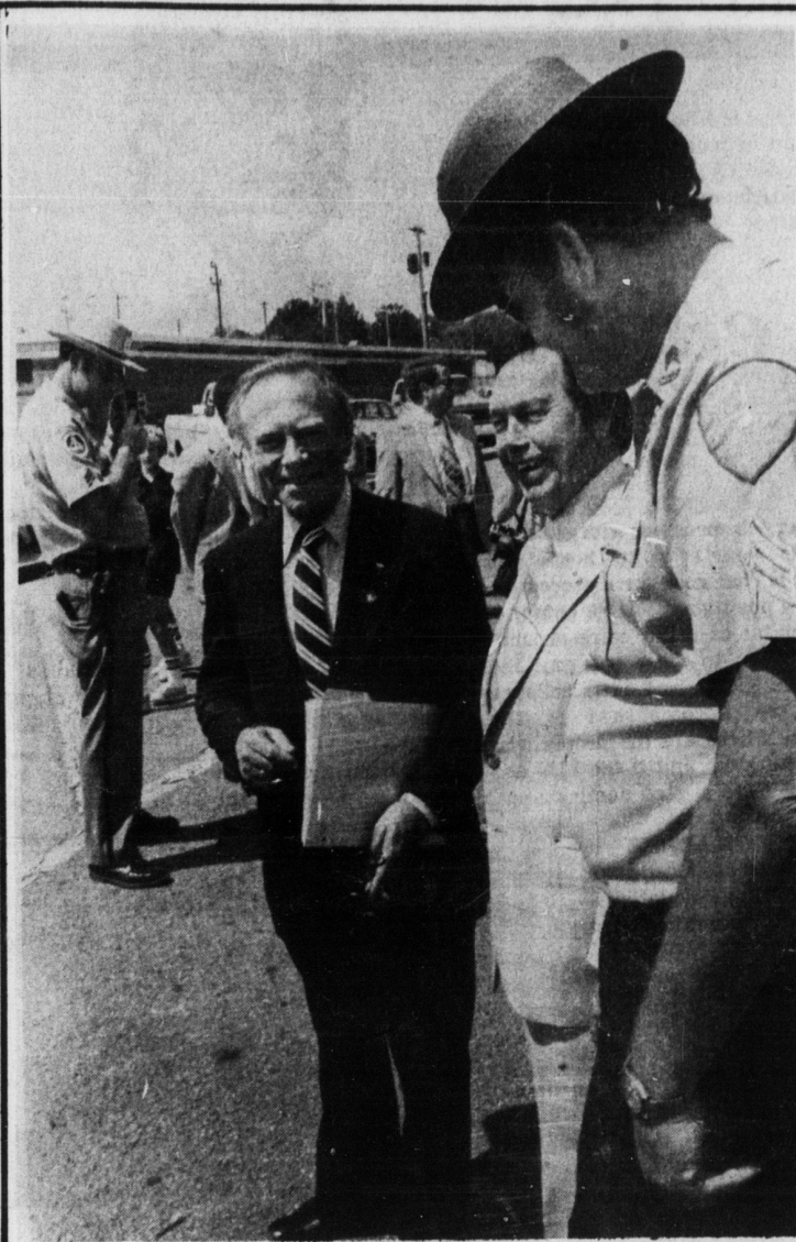
Photos by Tom McIntyre
