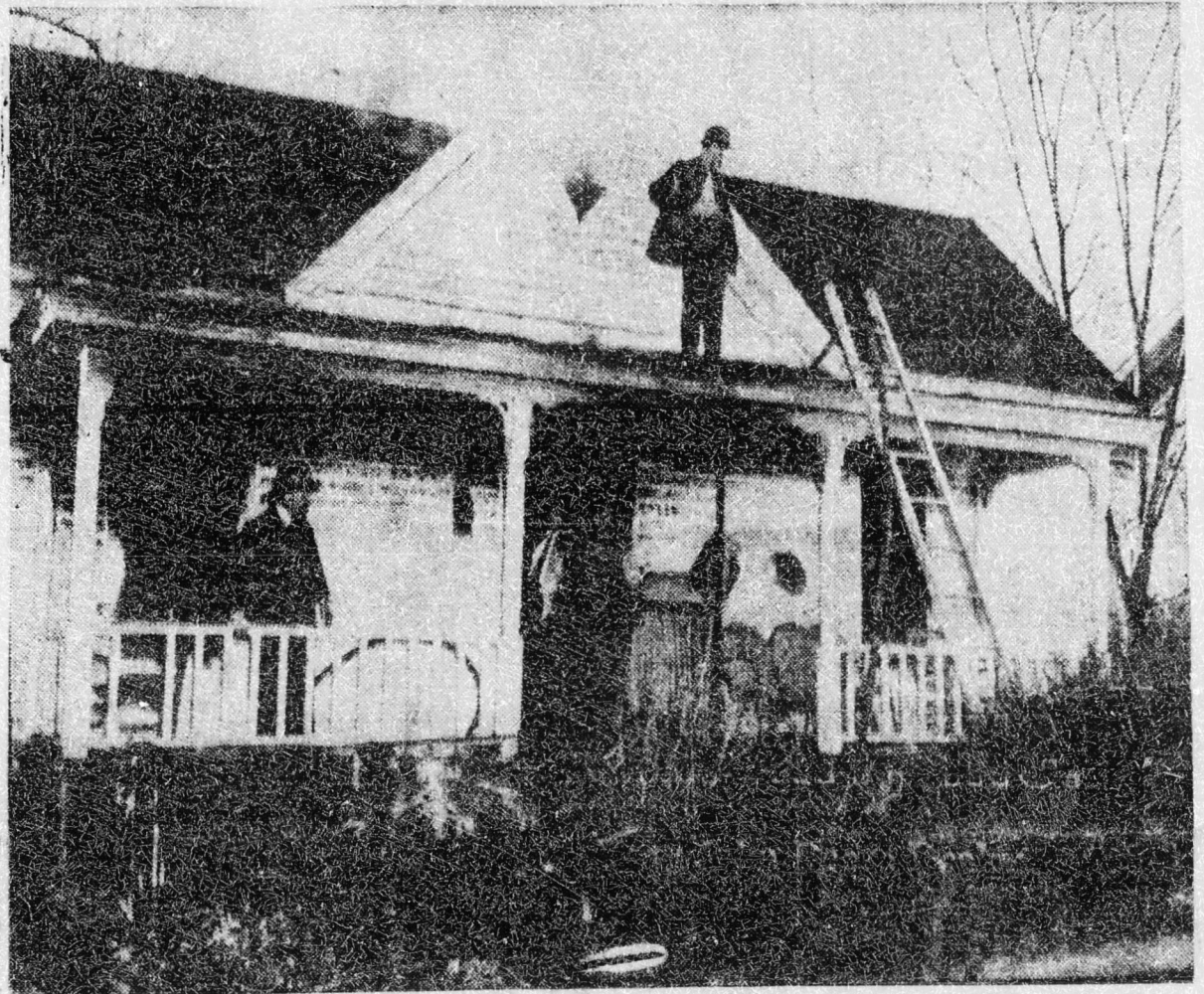
FIRE DAMAGES LOCAL HOME — Although no one was hurt when fire broke out at the above residence Monday at 2:45 p.m., considerable damage was done to the interior of the structure, located at 118 Camden Street. The origin of the blaze, which was confined to both the ceiling and the front portion, could not be ascertained. About 300 persons gathered to watch the firemen fight the blaze. (STAFF PHOTO BY CHAS. R. JONES).
