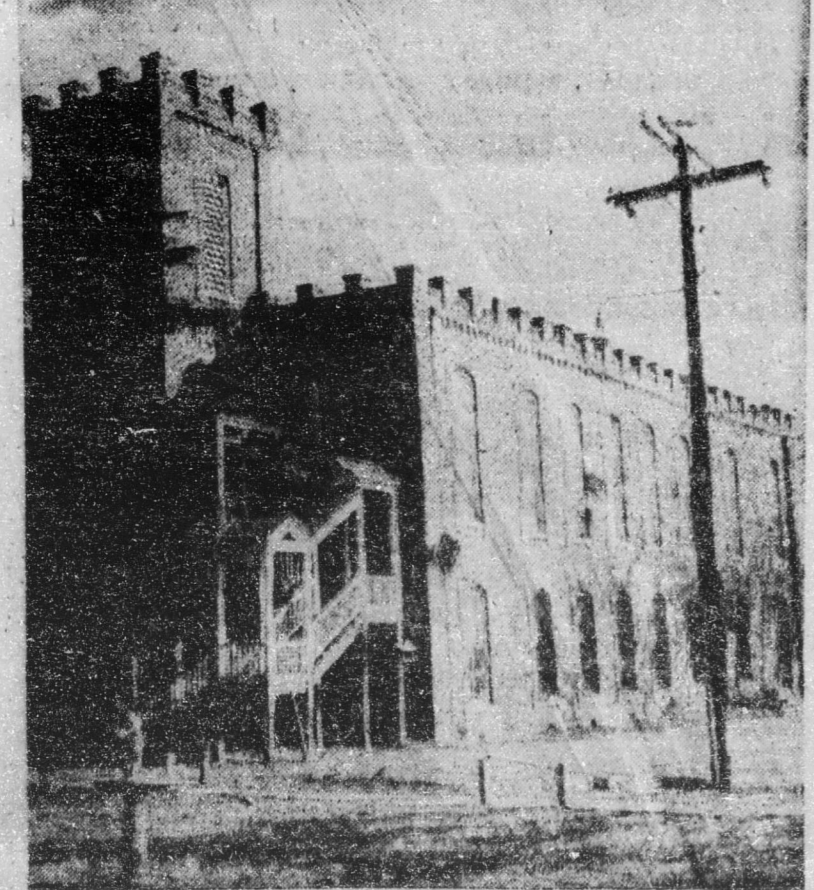
SHAW'S GREENLEAF AUDITORIUM CONDEMNED — The assembly hall at Shaw University, Greenleaf Auditorium, above, was condemned last weekend, according to Fire Chief Jack Keeter and Captain J. W. Holmes. It was reported that the condemnation followed attempts by the fire department to have the steps to the structure repaired and a back entrance provided in the event of an emergency. Some 450 students and faculty members had used the auditorium regularly. (STAFF PHOTO BY CHAS. R. JONES)
