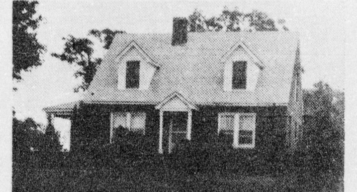
$243.20 for electricity for one year in the Hugh E. Barnette home on RFD 2, Roxboro. The Barnettes changed to an electric baseboard heating system for their 1,600 square foot home. Electric appliances include water heater, range, refrigerator, freezer.
