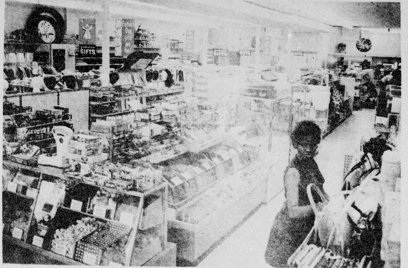
INTERIOR VIEW OF STORE
