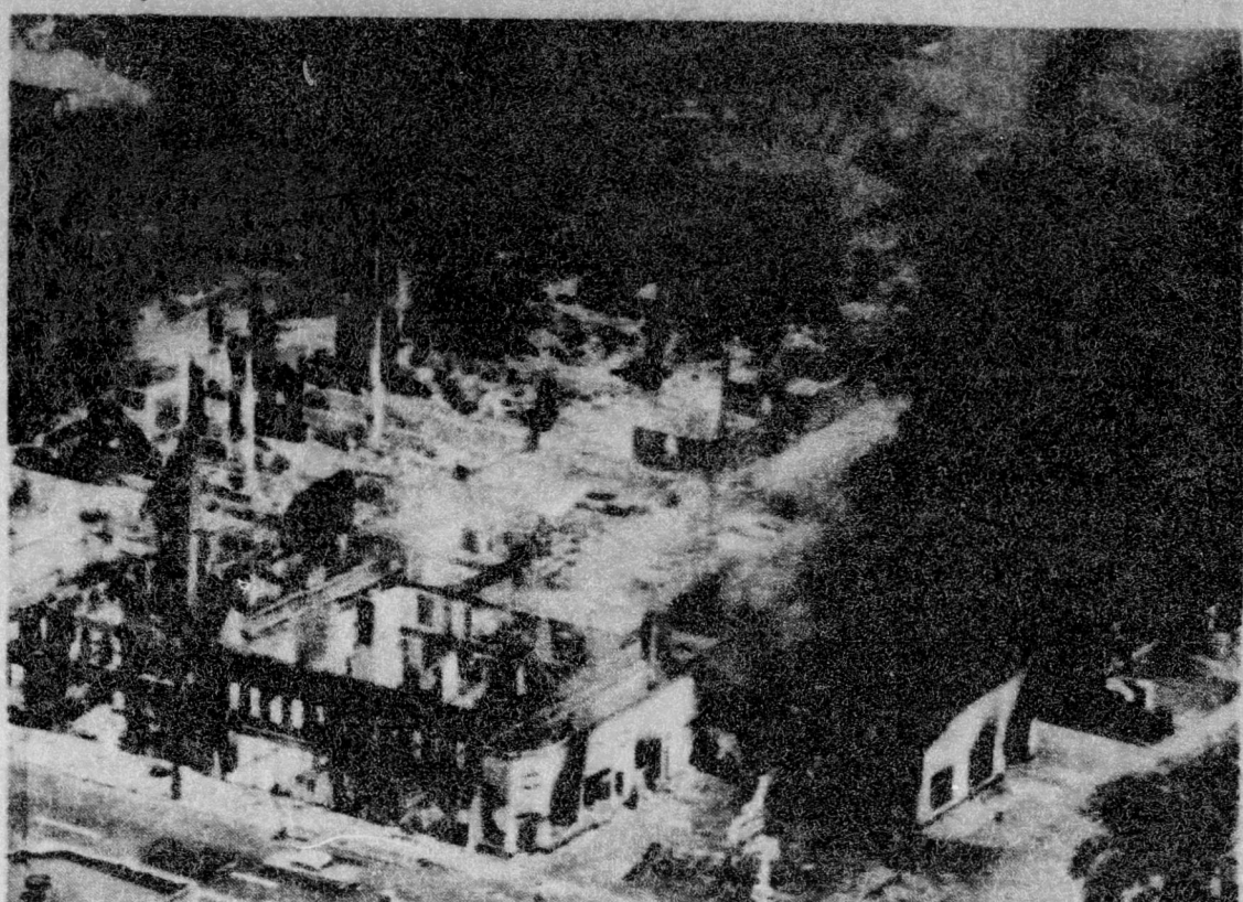
SCENE OF VIOLENCE - Detroit: The gutted remains of buildings (left) attest to the destruction caused by two days of rioting in Detroit's west side. A service station continues to burn (right) pouring smoke and flames onto other structures. At least 23 persons have been killed and more than a thousand injured in the two days of violence. (UPI PHOTO).
