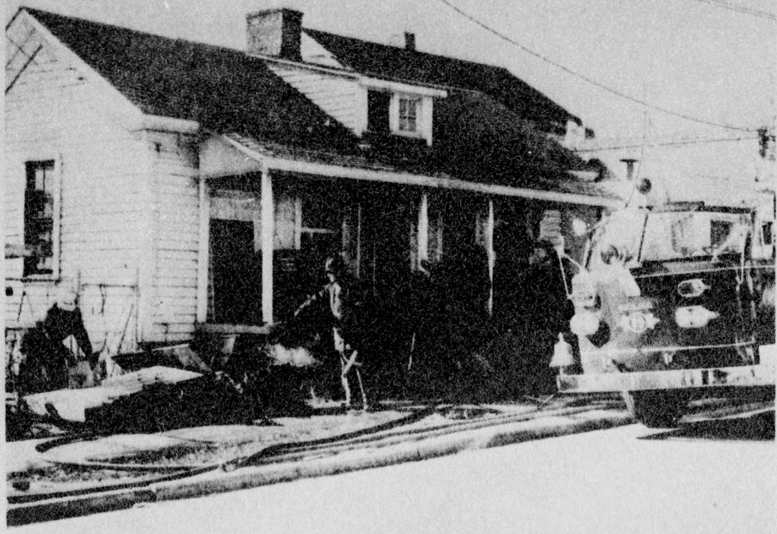
MARTIN STREET HOME BURNED - This picture shows the charred results of a fire which damaged the home of Mrs. Juanita McLean, 706 E. Martin St., Monday. The fire is said to have been caused by faulty wiring.
