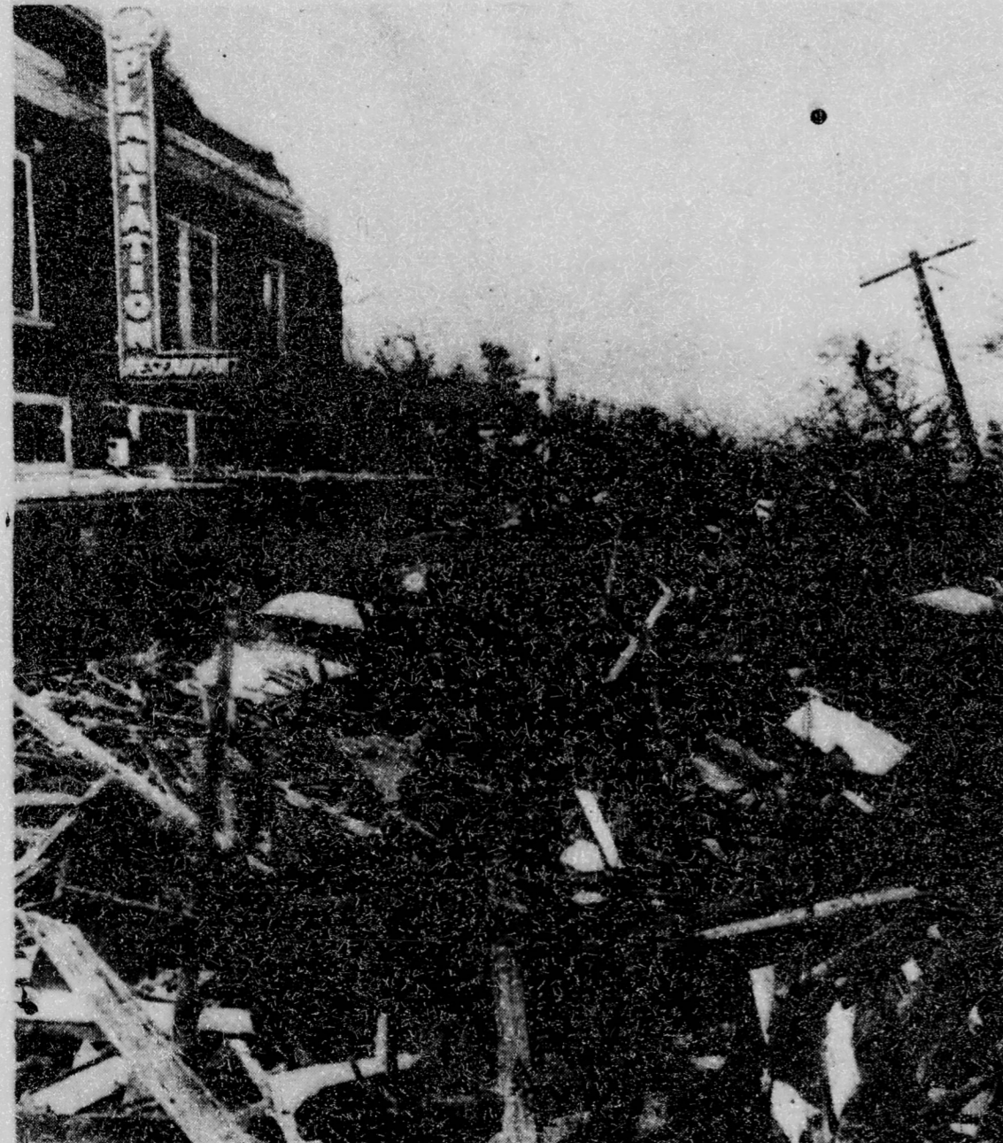
HURRICANE CAMILLE WAS HERE - Pass Christian, Miss.: Officials fear when rubble like this shown in downtown Pass Christian August 19 is cleared, many more bodies will be found. The rising death toll made Camille the biggest killer in more than a decade, since Hurricane Audrey left 430 dead in Texas and Louisiana in 1957. (UPI).
