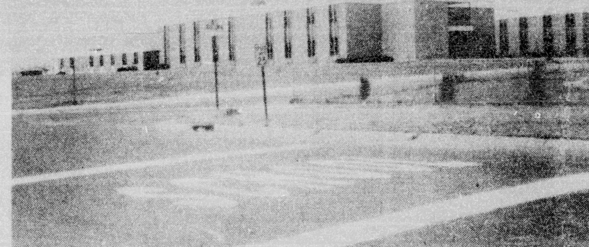
NEW DILLARD HIGH SCHOOL - Pictured here is the new Dillard High School in Goldsboro, standing in all of its splendor. The old school, located in a completely black neighborhood, is now situated some distance from its former location. The old school was gutted by fire.
