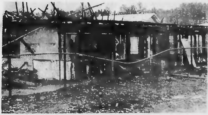
APOLLO HEIGHTS COMMUNITY CENTER BURNS — Shown above is the gutted remains of the Apollo Heights Community Center, located on Lunar Drive, which was destroyed by a mysterious fire early Sunday. Firemen suspect arson. See story. (Staff Photo).
