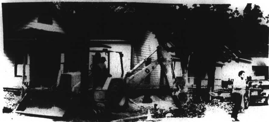
AREA DEVELOPMENT—These houses under construction on East Martin and East Streets are signs of community improvement and revitalization of the area. As downtown Raleigh expands, dilapidated, unkept businesses and homes that do not harmonize with the projected appearance scheme of the area must go. (Photo by James Giles, Sr.)
