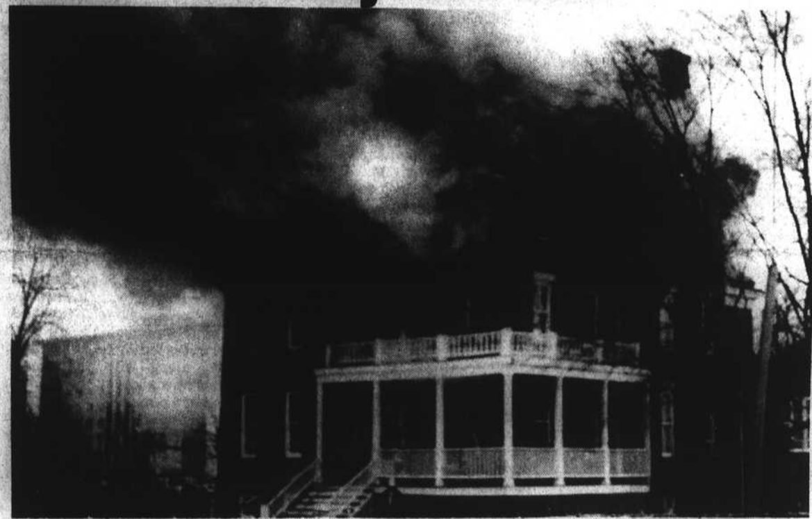
SHAW FIRE —One of the oldest buildings on Shaw University's campus, Meserve Hall, was gutted by fire last week displacing female students and leaving administrative offices damaged. Fire investigators had no estimates to the amount of damage to the 3-story structure which had been recently refurbished. (Photo by Patrick Elliott)
