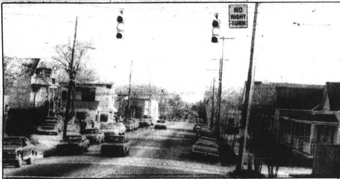
REDEVELOPMENT IN PROGRESS —The 200-400 blocks of S. East Street will continue redevelopment in conjunction with the City's Downtown East and the Thompson-Lucille Hunter School Redevelopment Plan. Pictured right are new single-family housing recently constructed. Pictured left are businesses and tenant housing that will be renovated or demolished for continued
