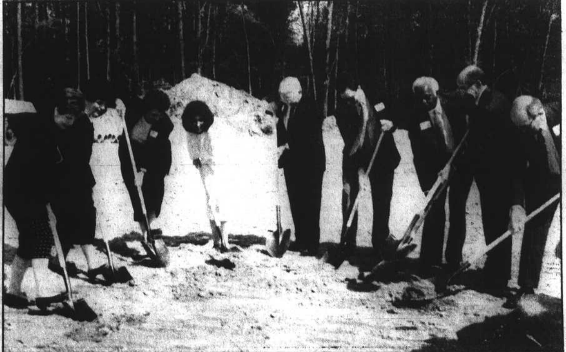
NEW HEALTH CENTER —A groundbreaking ceremony was held recently for the Alice Aycock Poe Center, located in Southeast Raleigh on Sunnybrook Road. The center, scheduled to open in 1991, will be a teaching facility where master teachers present courses in general health, nutrition, substance abuse, family life education and dental health. Pictured left to right are: Patricia R. Hackney, Shirley D. Lucey, Paula Hudson Hildebrand, Virginia M. Scanlan, Josiah R. Whitehead, Clark Smith, Vernon Malone, Edwin W. Monroe, MD and Thomas B. Dameron, Jr., MD.
