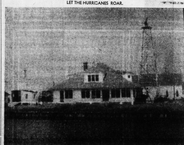
HERE at the right of the picture is the newly completed radar tower of the Hurricane Warning Center in process of activation by the U. S. Weather Bureau at Hatteras. So sensitive is the antenna perched at the top of the 65-foot tower that "it can see a duck landing on the water five miles away." It can also reach out into the center of a hurricane 300 miles away and take its secrets-its velocity, direction, and the power of its winds.
