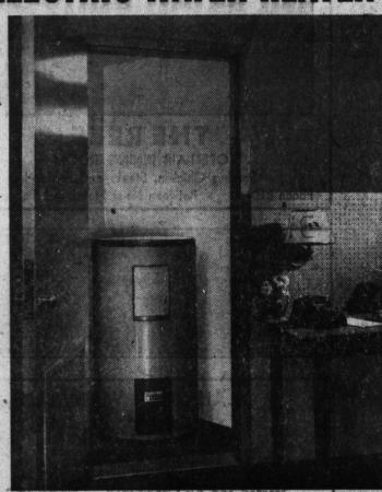
SO SMALL, safe, silent, automatic, that you can tuck it away in a closet and forget it. Needs no flue or vent. Gives off no heat, cool to touch all over.
