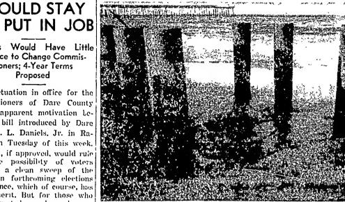
PILINGS AND PIPE have been combined in this project at Nags Head, which was installed last spring and summer as a matter of drain for water standing in areas between the old and new highways. It has served its original purpose with a good the proposed legislation is ap- degree of efficiency, but in addition has proved itself effective in stabilizing and building the beach. It is located east of the town office's former location, for all who came to take a look at it.
