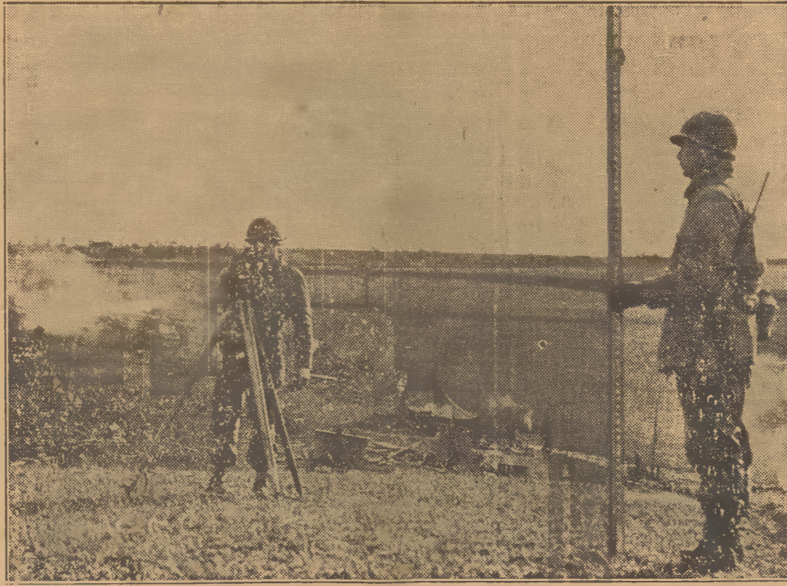
Released by U. S. War Department, Bureau of Public Relations. NINTH AVIATION ENGINEERS UNDER FIRE —While artillery pounds away at the enemy—note smoke from gun on left—men of the 922nd Engineer Aviation Regiment survey German field for new airstrip. T/Sgt. Shannon K. Dean, Ironton, Ohio, at the transit. Cpl. Alfred H. Gore, Brownfield, Texas, is rodman. (Official 9th AF photo.)
